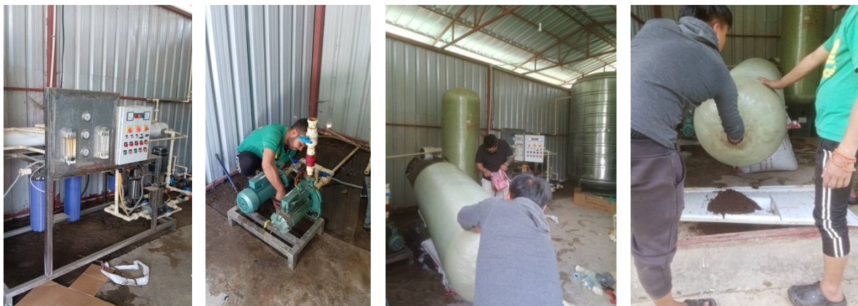
Figure 36: Picture showing the repair and maintenance of RO plant at NCAH
